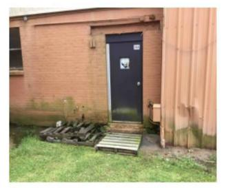
Draining is poor at between clasroom wings. Metal panel bent in various locations. Door stoop missing.
