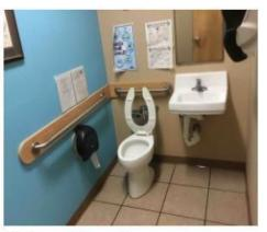
Restroom fixture clearances noncompliant, missing pipe insulation under sinks, door hardware noncompliant, door clearances noncompliant, typical throughout.
