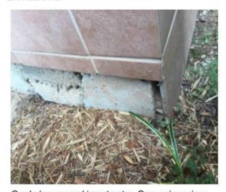
Grade beam cracking at entry. Occurs in various locations at building perimeter.
