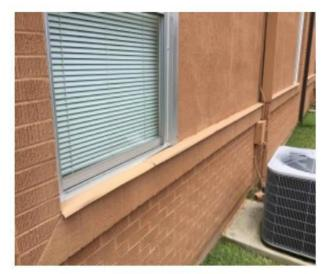
Metal window flashing along north façade is bent. Single pane windows and frames are in poor condition.
