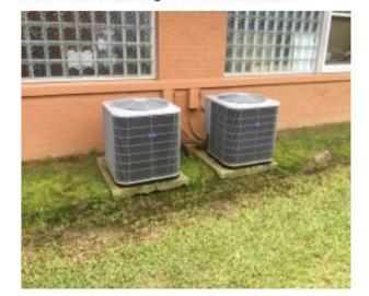
Erosion present at mechanical pads
