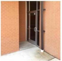
Door into courtyard does not have proper maneuvering clearance
