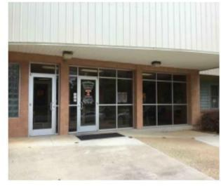
Tile cladding chipping at base. Metal soffit and fascia in fair condition. Soffit lighting is outdated. Storefront entry in good condition.
